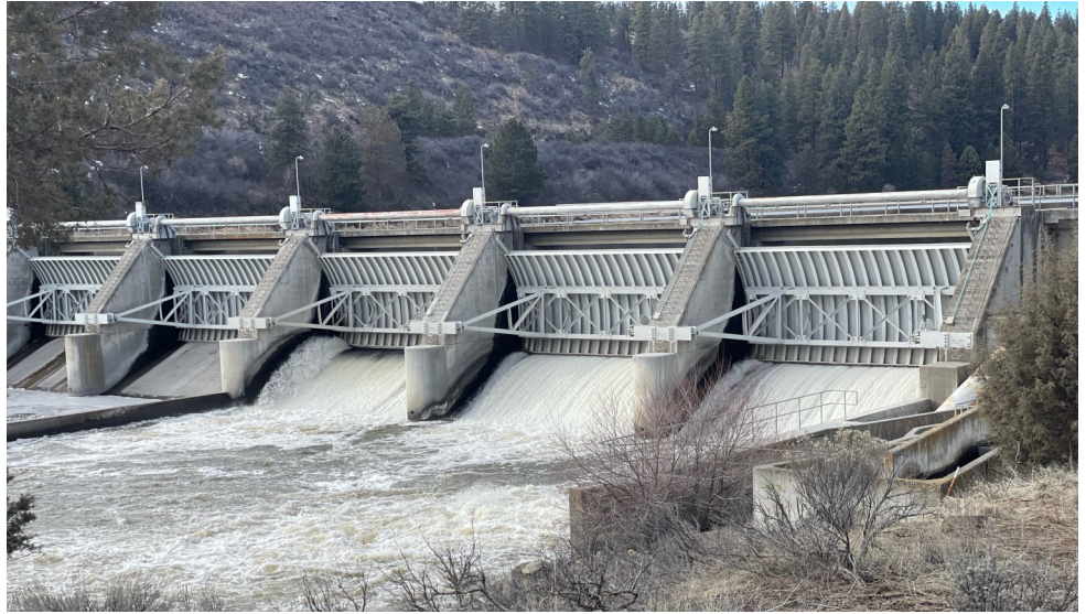
Keno Dam Feb 8, 2023 Photo by Kellianne Sites
