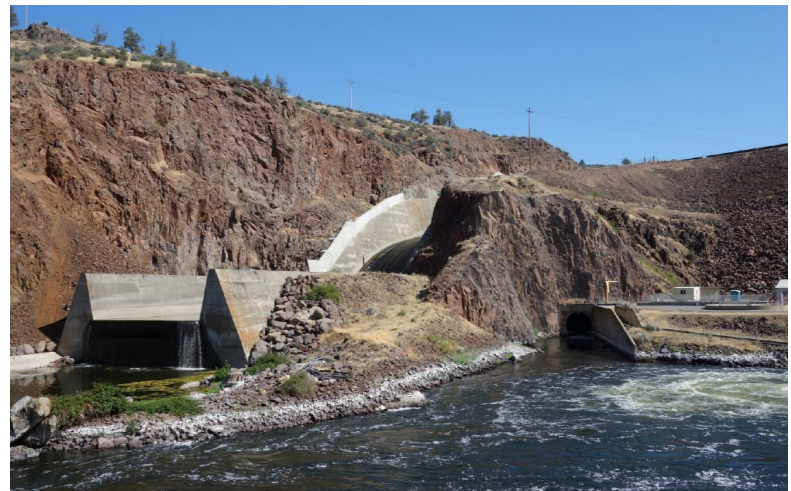
Iron Gate Dam spillway and diversion tunnel. Image courtesy of KRRC.
