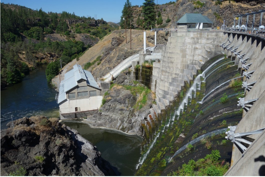
Copco 1 powerhouse as seen from the top of Copco Dam. Image courtesy of KRRC.
