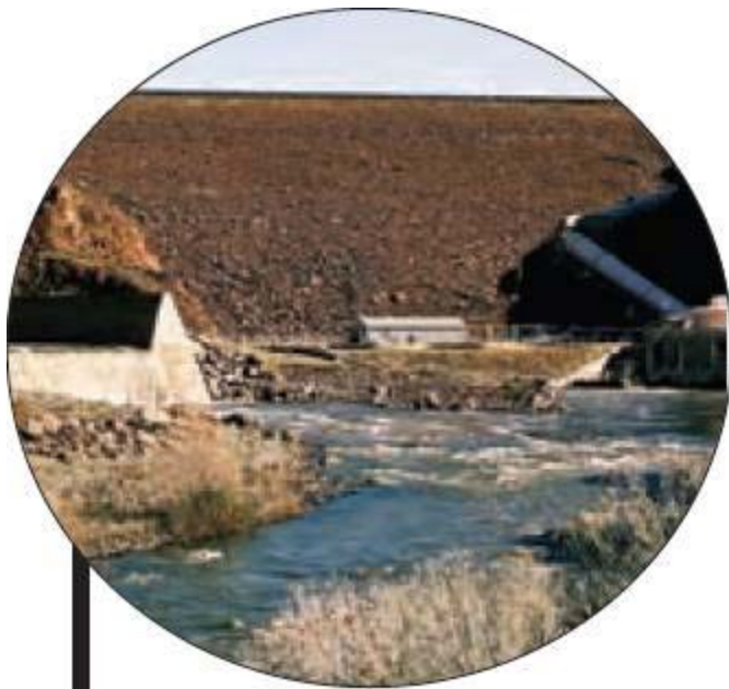
Iron Gate Dam
