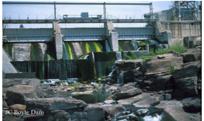
JC Boyle Dam on the Klamath River in Oregon
